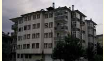
Safranbolu, Akkonut Sitesi MGK 300x1 adet (296 kW)
