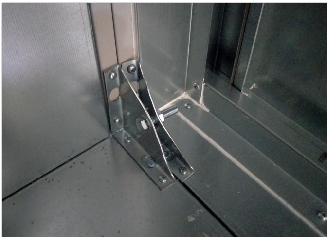
Fig. 16. Corner connection
