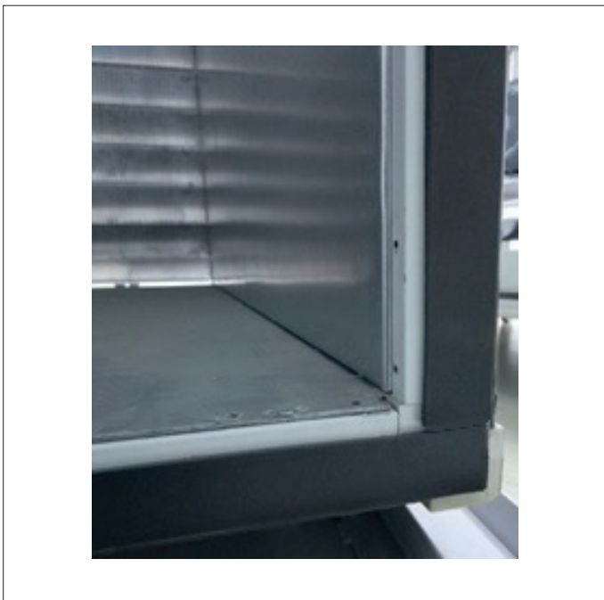
Fig. 20. Insulation tape application
