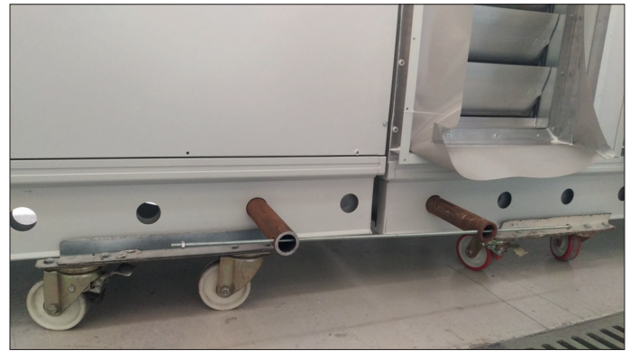
Fig. 12. Connecting the sections using threaded bars
