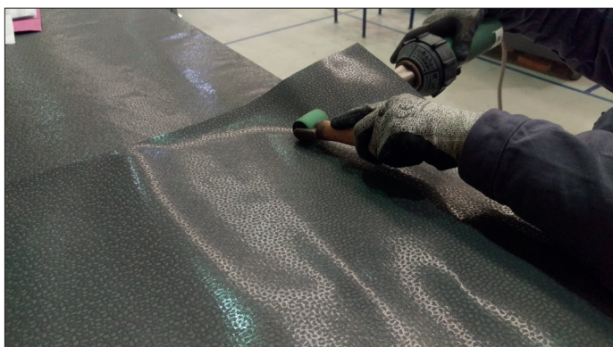
Fig. 47. Roof installation, method 1
