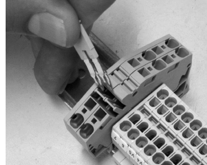
Remove shunt to deactivate a heater (reduction of 300w)
