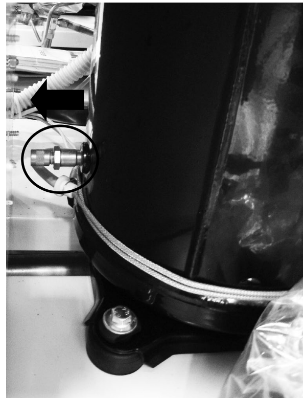
Shift the electric box to allow access to the oil level gauge.
