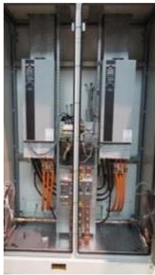
Frequency converters compressor drives + main power connection
