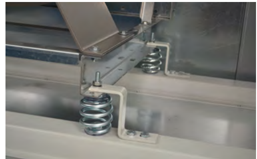
Spring anti vibration mounts
