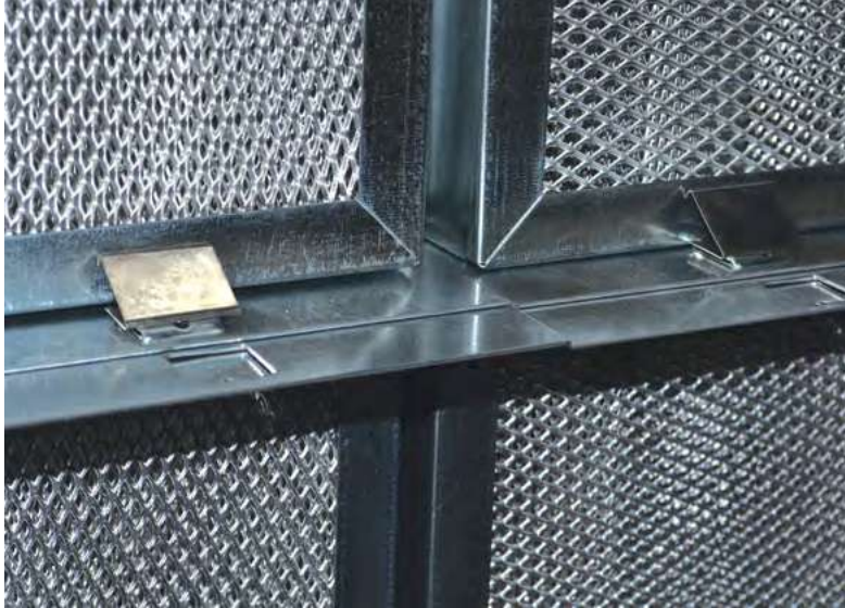
Tightening clip for front withdrawable filter
