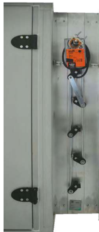
Damper movement mechanism
