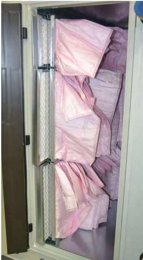
Side withdrawable combined filter (panel + bag)
