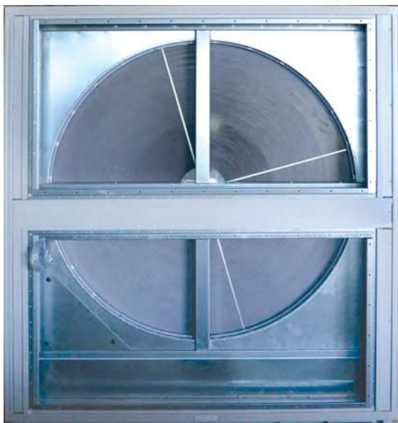
Wheel type heat recovery
