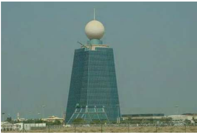
Etisalat Data Center, Fujairah - UAE
