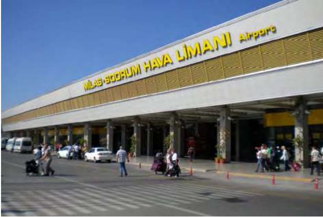
Bodrum Airport - Muğla
