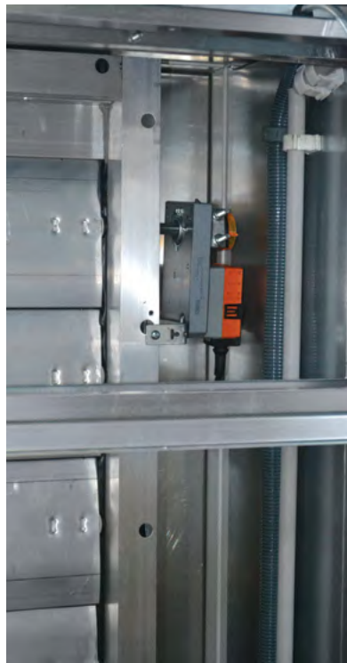
Internal or external damper actuator
